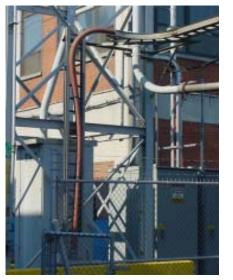
Figure 2. Outdoor metal clad cable in cable tray.
