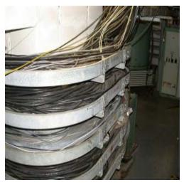
Figure 6. Overloaded Cable Tray.
